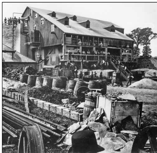
Figure 12. The crushing mills, known as the High Level at Mountsorrel Quarry, with curious workforce looking on, c1880. The barrels are filled with crushed granite, ready for distribution. (Photo: Lafarge Aggregates)
