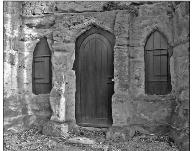
The cave from the outside with its new doors and shutters.
