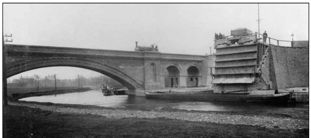
Figure 13. The bridge at Mountsorrel, c 1870, with a locomotive on it. Right of the bridge are the loading chutes, with side-tip wagons on top feeding aggregate to barges on the canal. (Photo: Lafarge Aggregates)
