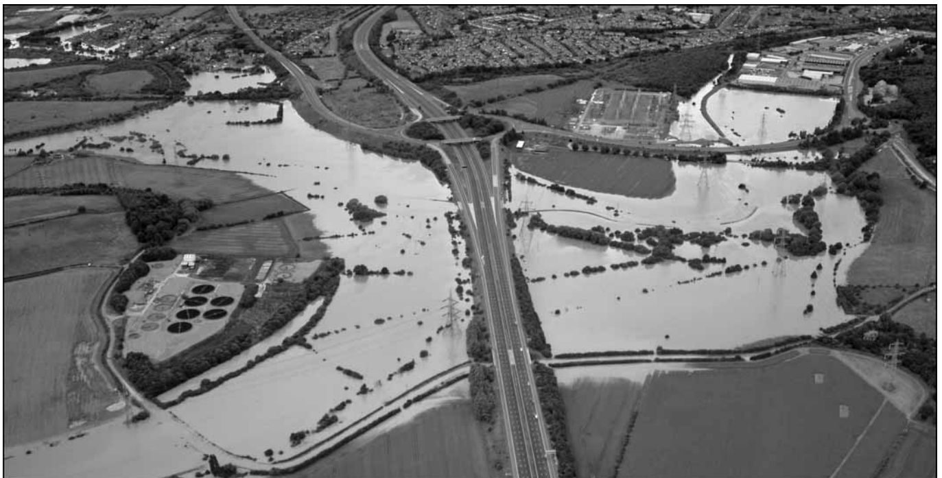
Active floodplain of the River Rother, with backflooding into Catcliffe village (top left), beneath junction 33 on the M1.
