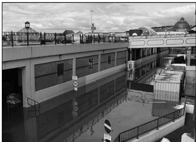
Floodwater in the Meadowhall Centre.
