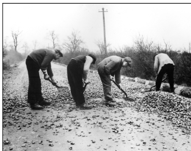
Figure 3. Manually laying a road, Mountsorrel. Date unknown. (Photo: Lafarge Aggregates)
